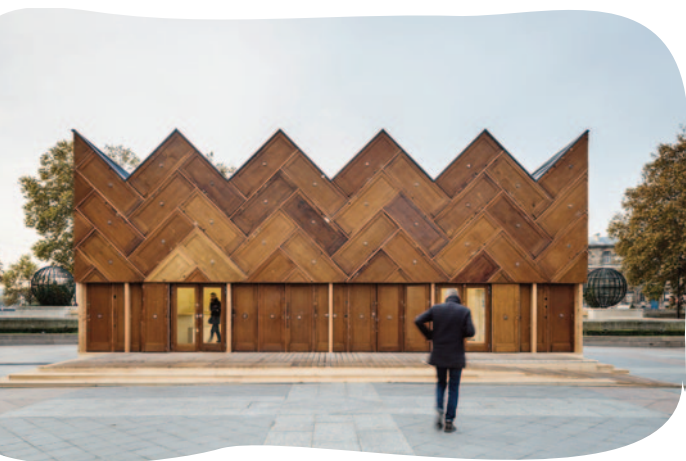
Circular pavilion, Encore Heureux, photographers: Cyrus Cornut + Florence Morisson (construction site)
